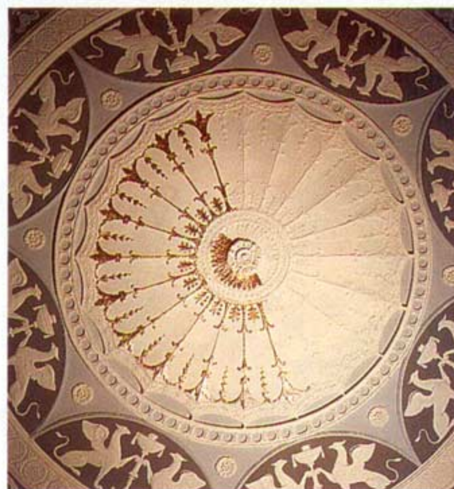
Eight pairs of griffins surround the 6½-foot-diameter ceiling medallion of Savannah's Lucas Theatre. All the plaster ornaments in the theater were restored by Jean-François Furieri.
